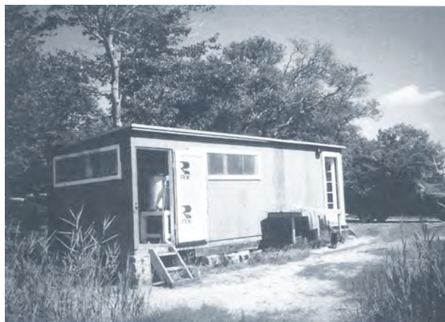
Hatchery facility at Island Pond.
